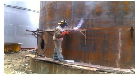
Tank fabrication and erection
